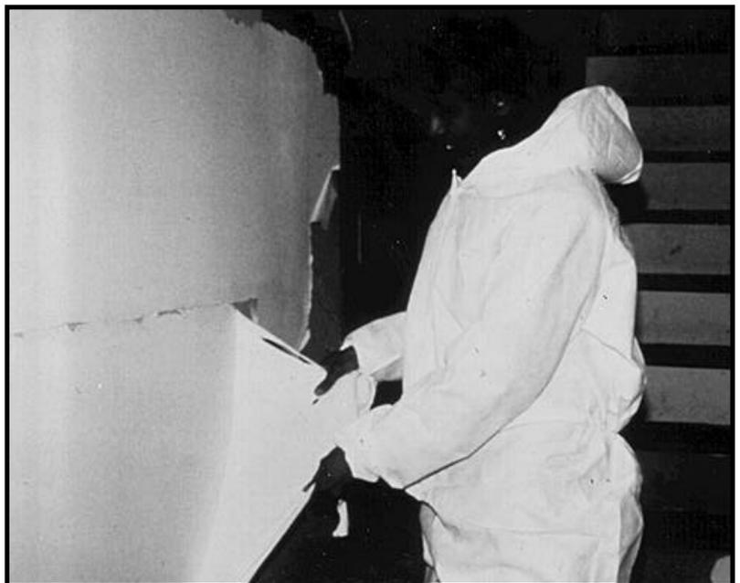
Figure 13.1 Encapsulant Failure.
